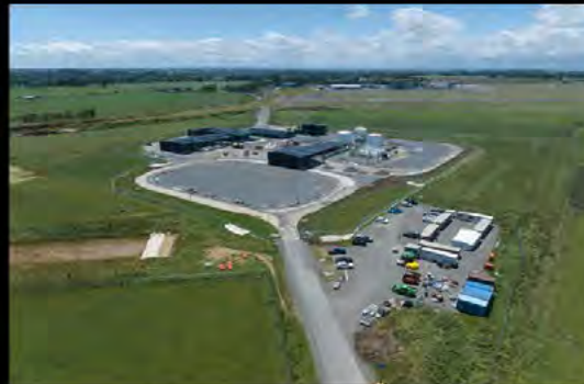
Aviation Fuel Installation at RNZAF Base Ohakea
