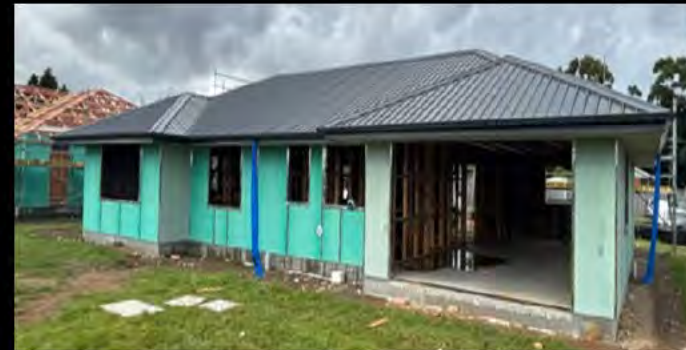
New housing construction at Linton Military Camp
