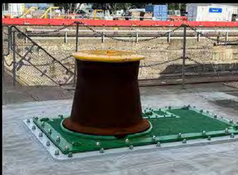
Dry Dock Capstan Replacements, Devonport
