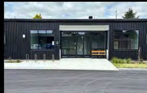
New Defence College Lecture Rooms, Burnham
