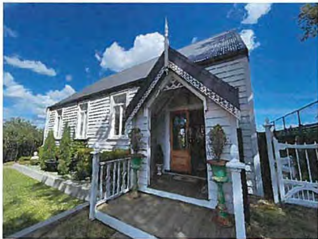
Exterior, Front Entrance
